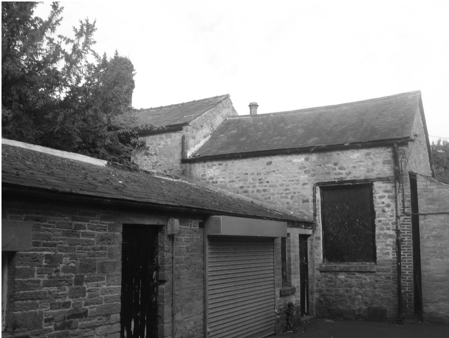
Structures to be demolished:
